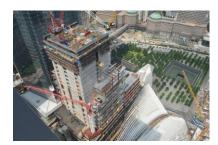
The first WOLFF in Manhattan: With the construction of the core always several floors higher up than the outer shell of 3 WTC, the WOLFF 700 B US (at the bottom) profits from a very short counter jib enabling it to rotate freely.
